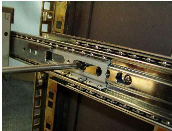
Figure 25: tighten internal slide rail screws
