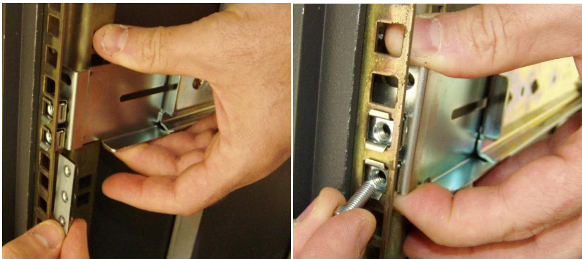
Figure 22 + 23: Slide rail attachment to rear ladder
